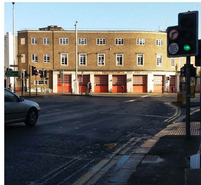
Preston Circus Fire Station, Brighton
